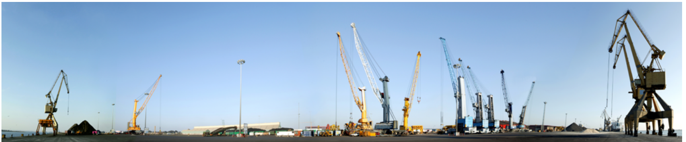
SEA-PORT BRIDGE CRANES
